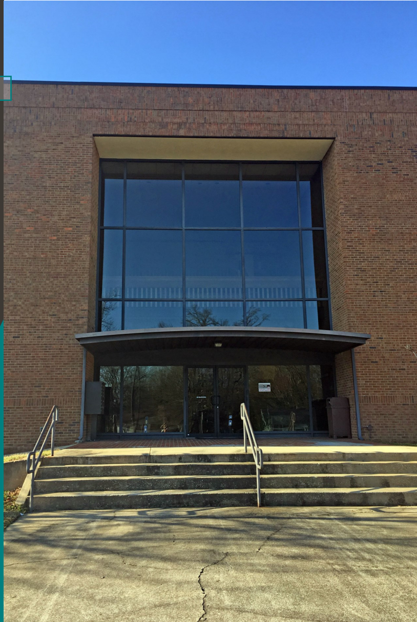
Side entrance, direct access to parking area
