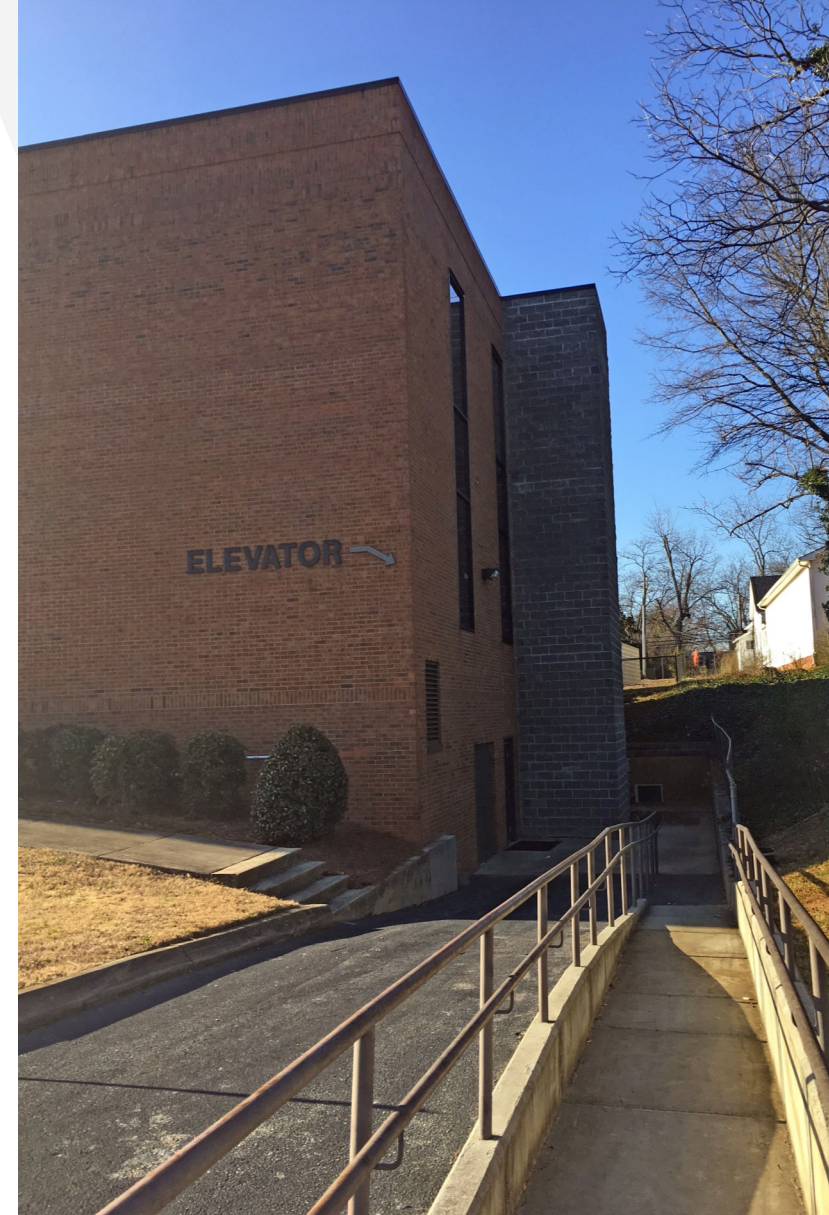
Building Elevator with ADA Access
